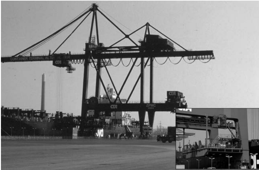
Figure 7.6 Separated crane functions, including a buffer (CTA Hamburg)
