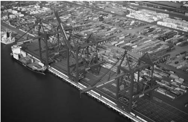
Figure 8.1 Terminal Burchardkai, HHLA, Hamburg, Germany
