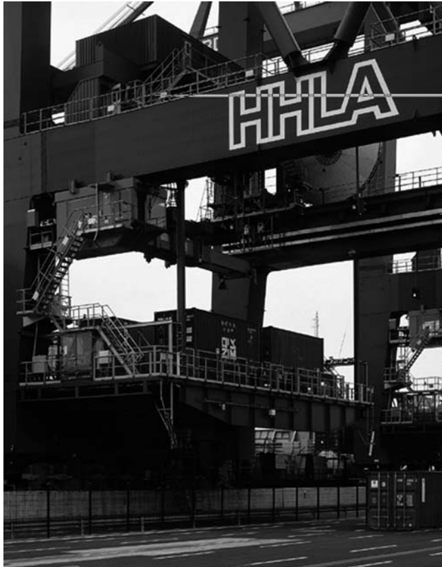
Figure 8.6 Lashing platform of one of the double trolley quay cranes at terminal Burchardkai, HHLA, Hamburg, Germany
