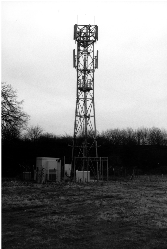
Figure 10.4 A typical cellular telecommunications base station along the roadside
