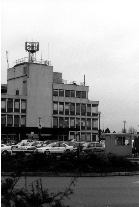
Figure 10.8 A typical cellular telecommunications base station located on a tall building covering an area of a town
