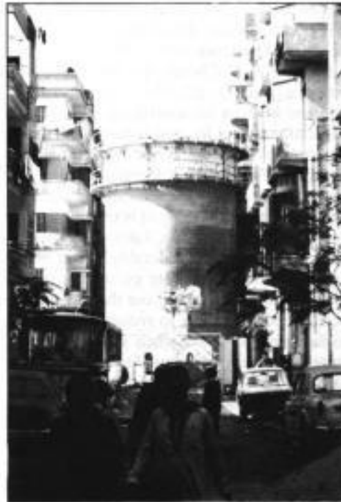
Fig. 10.34. Sinking of caisson in a narrow city street, Cairo waste water scheme (Flint et al. 31 )
