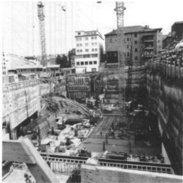
Fig. 4.33. Composite use of contiguous bored pile walls and gunited steel soldier beams retained by ground anchors, Stuttgart (courtesy of Bauer)
