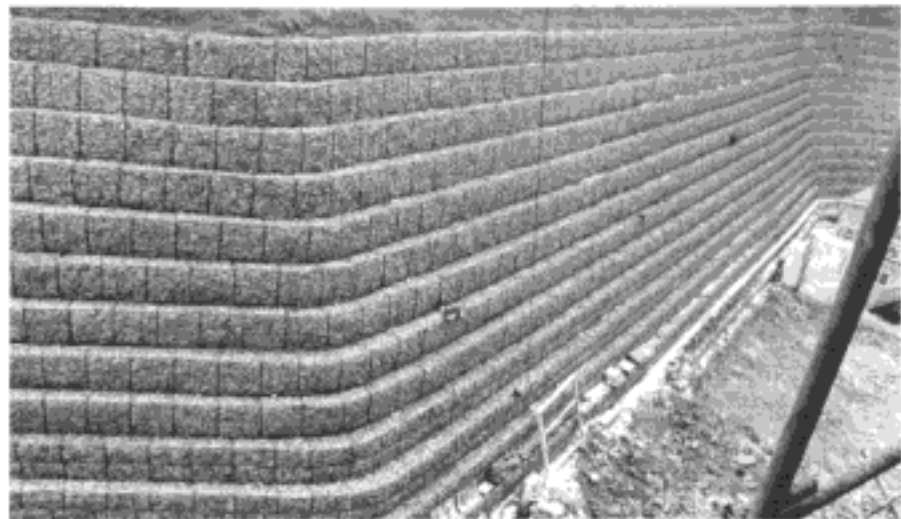
Fig. 3.19. Combined gabion box and reinforced soil system known as Terramesh: (a) vertical face; (b) stepped face; (c) with a hydroseeded face; (d) example of a stone-filled Terramesh wall in Taiwan (courtesy of Maccaferri)
