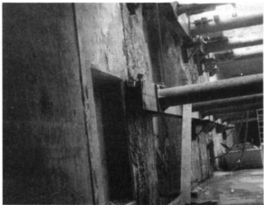
Fig. 9.28. Cairo Metro: junction between precast and in situ diaphragm walls
