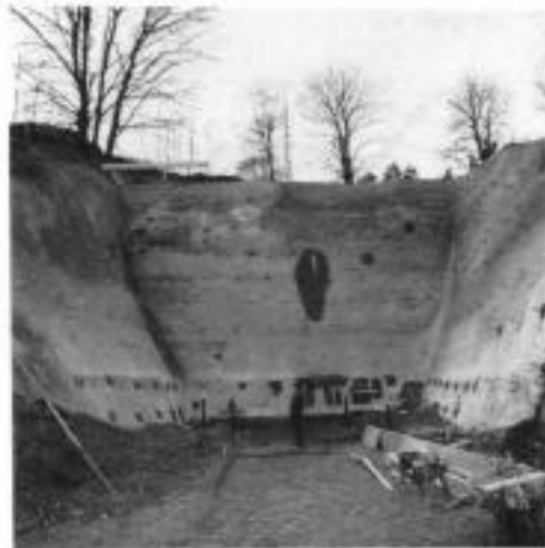
Fig. 8.3. Soil-nailed slope at Pocking, Bavaria (courtesy of Bauer)
