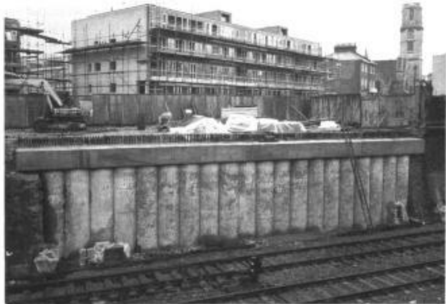
Fig. 4.15. Secant piles, Piccadilly Line underground railway, Heathrow Airport (courtesy of Lilley)
