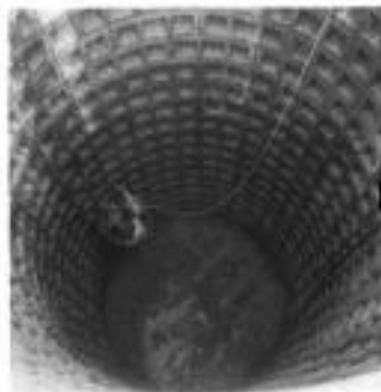
Fig. 10.3. Conventional bolted precast concrete segment lining (courtesy of Charcon)
