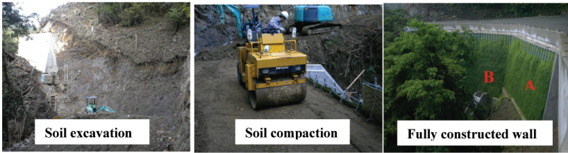
Photo 1. Construction of reinforced chain wall
