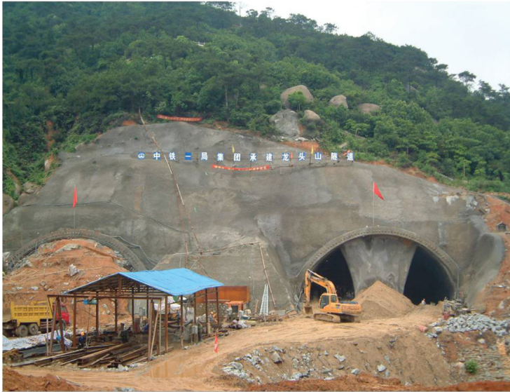
FIG. 1. Both side drift method of Longtoushan Tunnel
