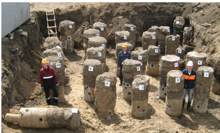
FIG. 6. Experimental jet-grouting columns.
