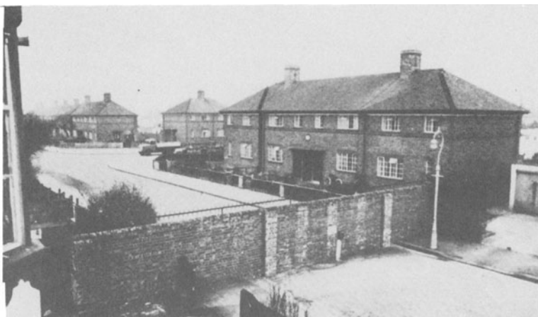
The wall in Carlton Road seen from the urban housing estate
