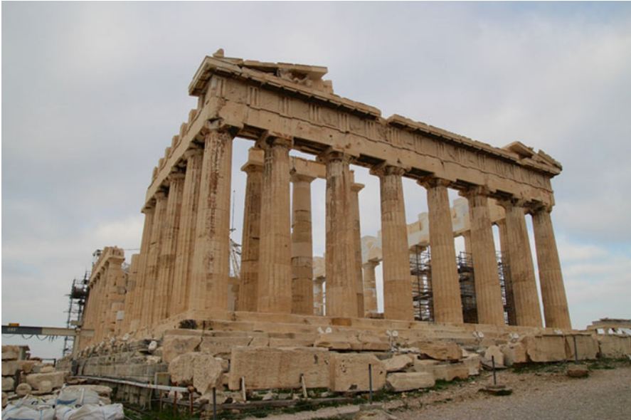
Fig. 5.3 West side of the Parthenon. Most parts of the pediment were destroyed during the Roman Empire period (Photo by T. Ohsumi)
