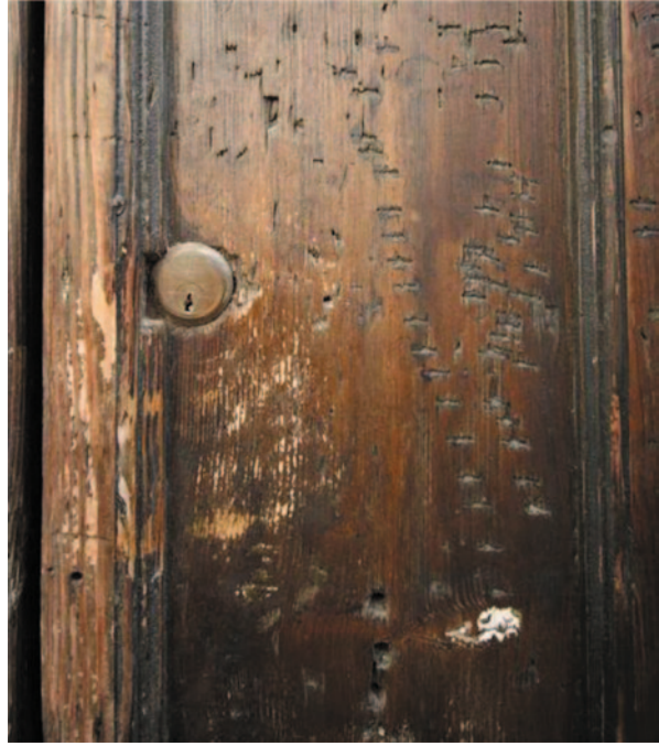
Fig. 15 Degradation by incisions, Venice
