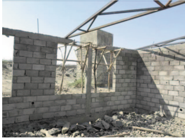
Fig. 4 Block construction, detail. (Photo by author)
