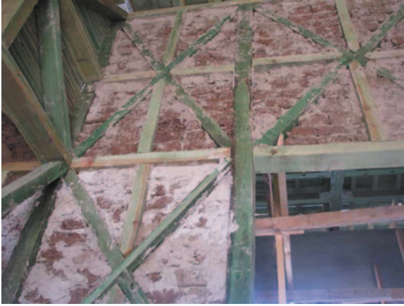
Fig. 7 The construction of the cob filled timber walls
