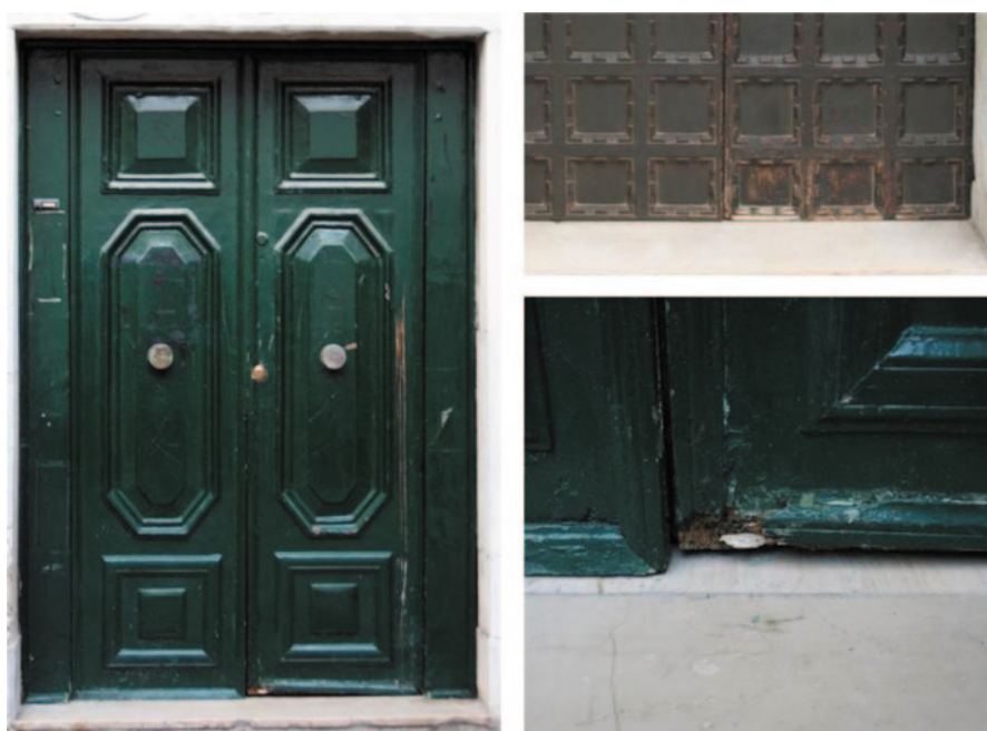
Fig. 9 Degradation by hitting, Venice
