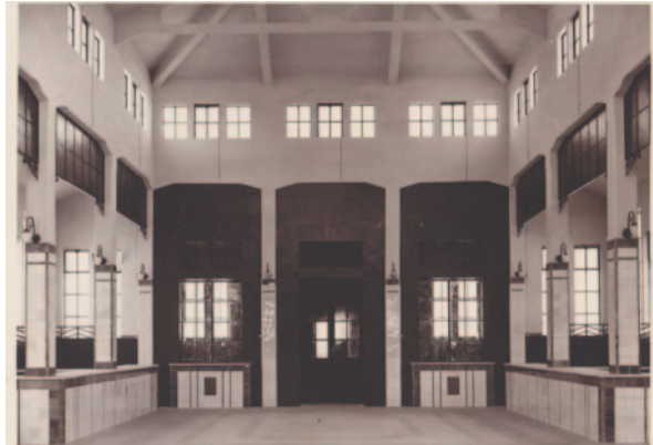
Fig. 2 The market hall interior. Private archive
