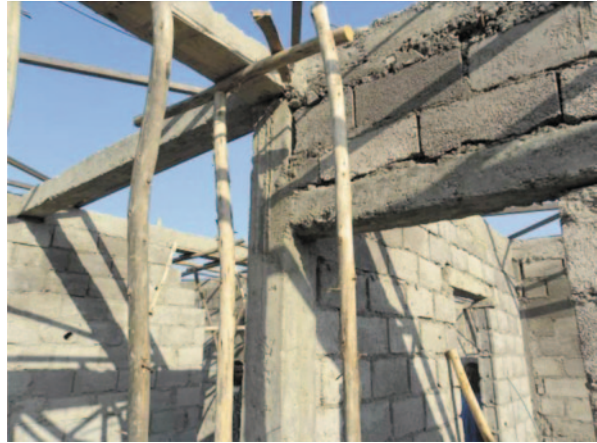
Fig. 2 Detail of concrete construction. (Photo by author)
