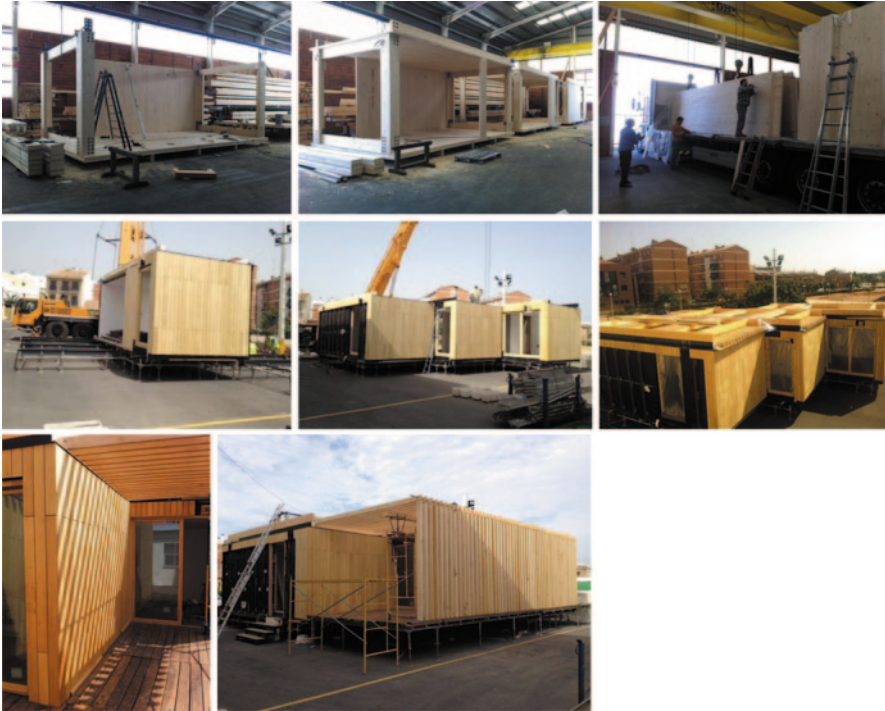
Fig. 4 Photos during the assembly of the SMLsystem modules
