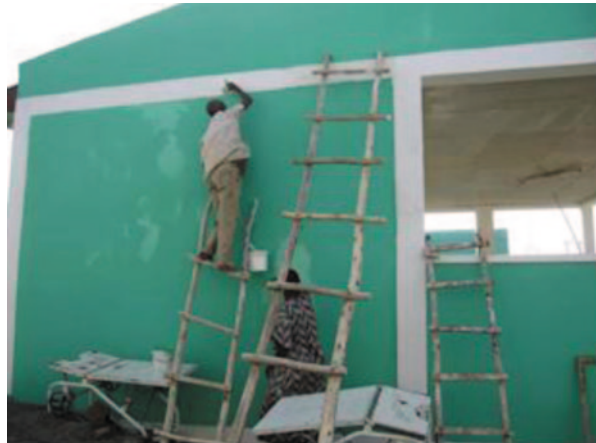
Fig. 7 Construction aids, ladders and scaffolding, in Assayta, Ethiopia. (Photo by author)
