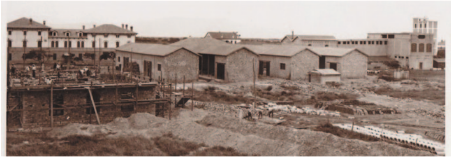
Fig. 1 The town hall under construction. Private archive
