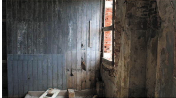
Fig. 7 Abandoned cloister without woodwork, Venice
