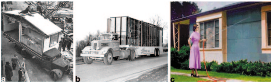
Fig. 4 a Truck transporting the house AIROH, 1945 [7]. b Truck transporting the house Lustron, 1948 [6]. c Exterior house Lustron [6]
