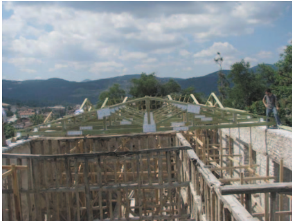
Fig. 6 Timber trusses constructed on the stone walls
