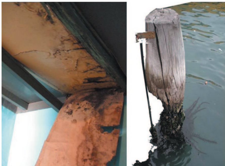
Fig. 12 Inadequate use of material, Dakhla ( left ) and Venice ( right )
