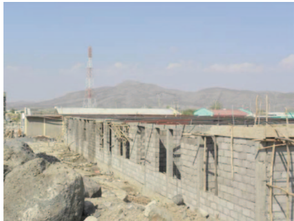
Fig. 5 Block construction, detail. (Photo by author)
