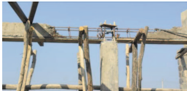
Fig. 3 Detail of concrete construction. (Photo by author)
