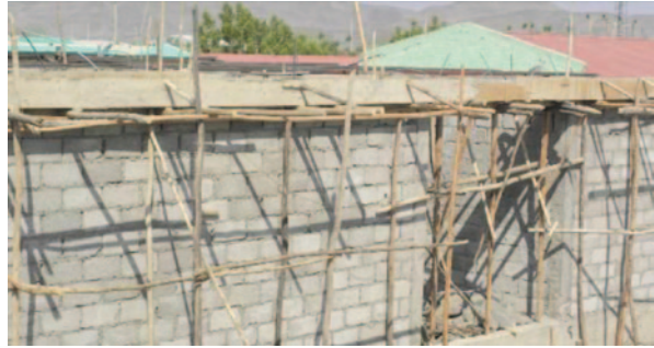
Fig. 8 Construction aids, scaffolding, in Assayta. Ethiopia. (Photo by author)
