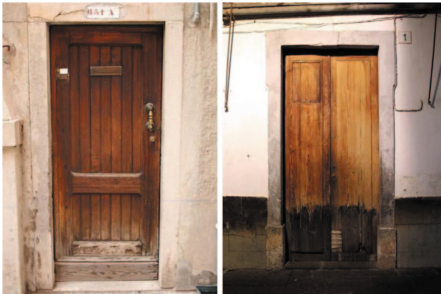
Fig. 3 Degradation in lower parts , Gran Canaria
