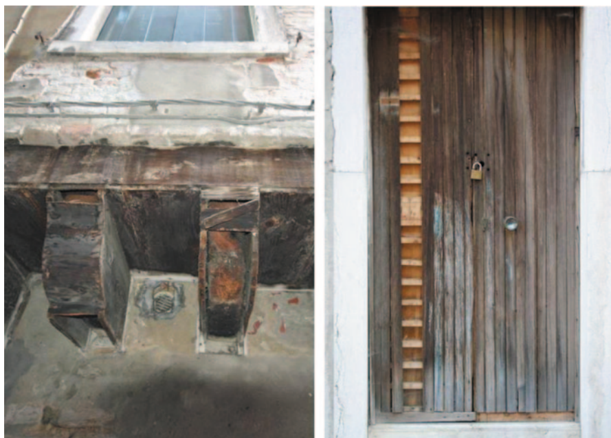
Fig. 13 Degradation by the thickness of the elements, Venice
