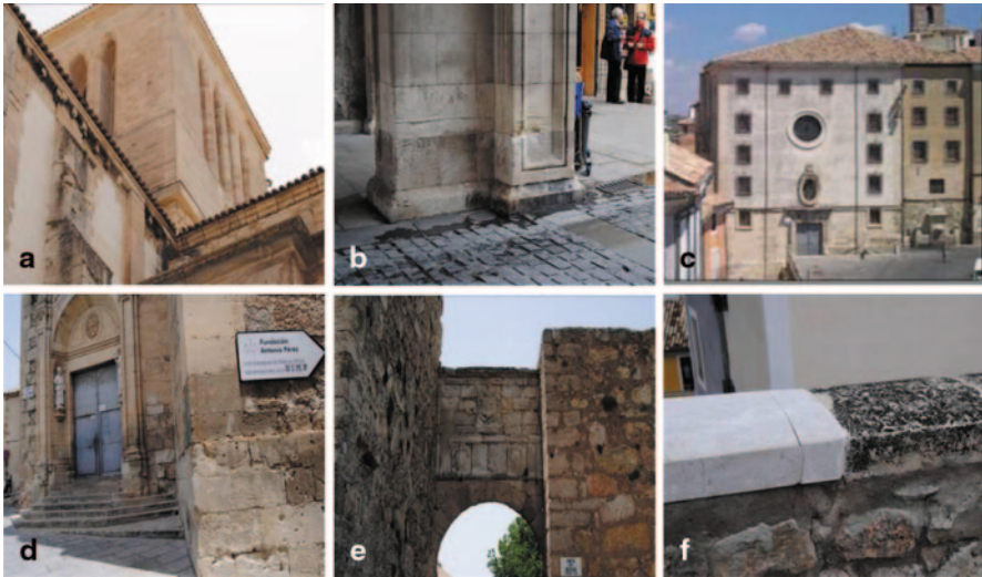
Fig. 2 Images of historic buildings in the city of Cuenca. A) Cathedral of Cuenca; lantern, cross, and flying buttresses of Arcos de la Cantera stone. B) City Hall of Cuenca; limestone pilaster, Júcar River quarries. C) Monastery of “Las Petras”; limestone quarries of the Júcar and Huécar rivers. D) St. Peter’s Church; limestone from Ciudad Encantada. E) Gateway to the castle; the arches are made of stone from Ciudad Encantada and the badge is made with stone from Arcos de la Cantera. F) Replacing part of the top of the wall (Ciudad Encantada limestone—right) with Vara del rey limestone (left in photo)
