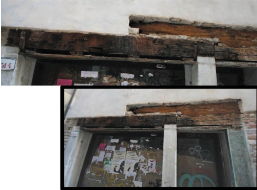
Fig. 19 Degradation by surface tension, Venice
