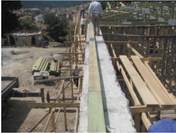
Fig. 5 The timber beam for supporting the trusses on stone walls
