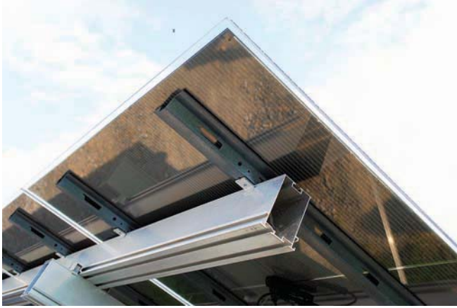
FIG. 17—PV module with mounting rails fixed to the back of the module with adhesive.
