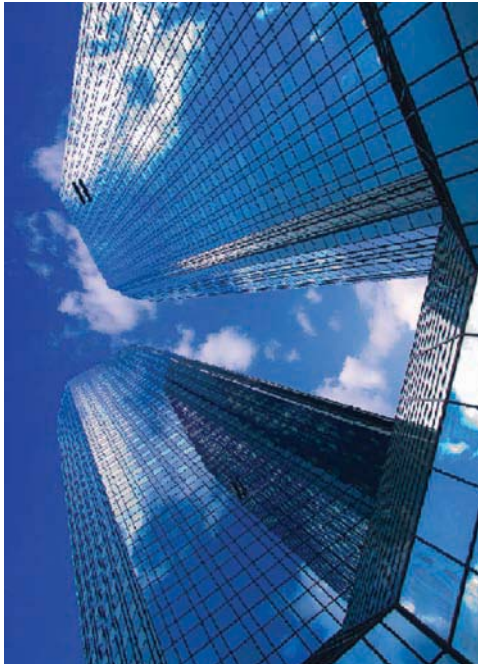
FIG. 1—Skyscraper – structural glazing with insulating glass.
