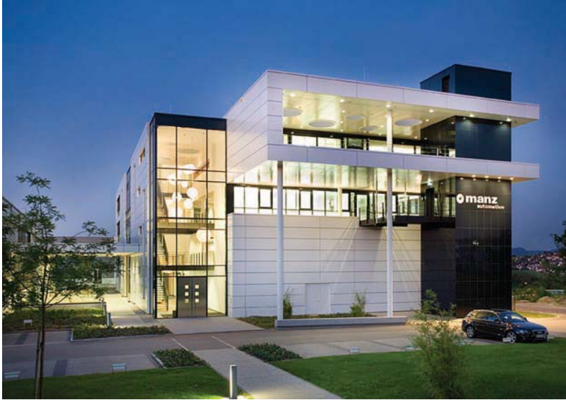
FIG. 20—Bonded Photovoltaic system facade, Manz Automation, Reutlingen, Germany (Hank und Hirth Freie Architekten; photo: Oliver Starke).
