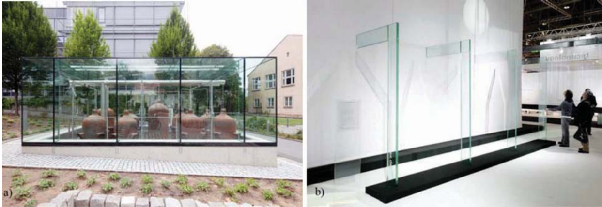
FIG. 2—Transparently bonded glass frames: (a) all-glass enclosure at the IFW in Dresden, and (b) prototypes at glasstec 2010 in Düsseldorf.
