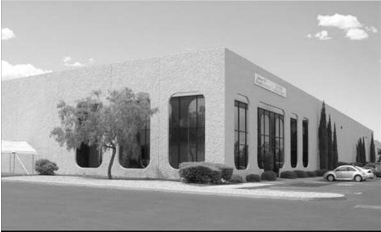
FIG. 1—El Paso, TX, tilt-up warehouse used for exposure of high performance acrylic and polyurethane sealants.
