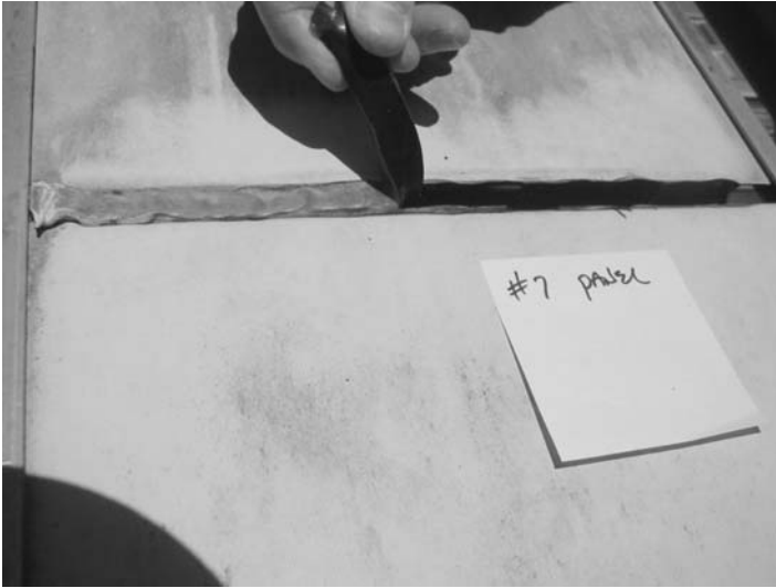
FIG. 23—Silicone sealant #7, after cleaning.
