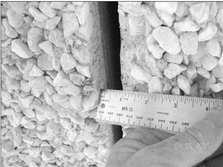
FIG. 2—Example of a prepared joint 1 in. (25 mm) wide. The underlying concrete slab and exposed aggregate surface layer are readily visible.
