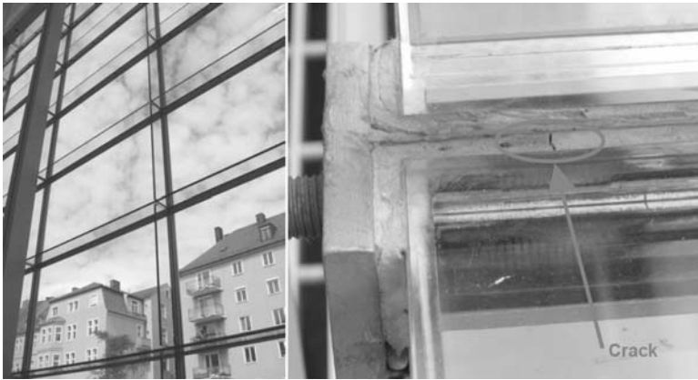
FIG. 3—Glass façade in the year 2008.
