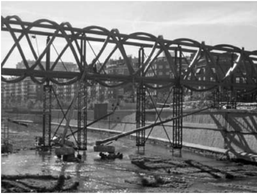
Figure 21. Propped footbridge over the river.
