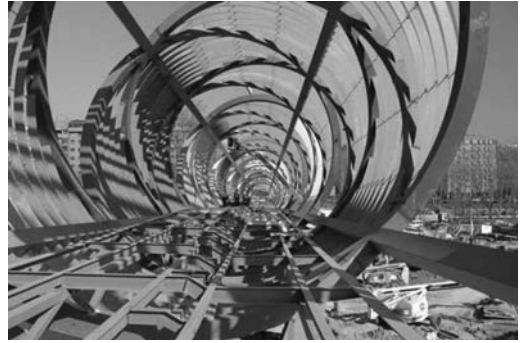
Figure 8. Deck substructure under construction. Notice the two lanes—pedestrian, bicycle—with different slopes.
