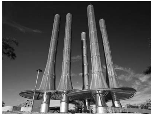
Figure 1. Image of the five Chimneys.
