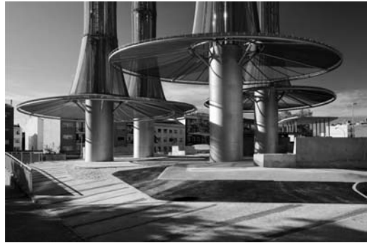
Figure 17. Two chimneys are joined by a canopy.
