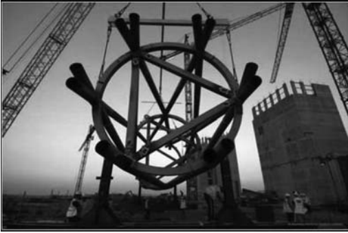
Figure 12. Arch assembly: Sub units being lifted into position.
