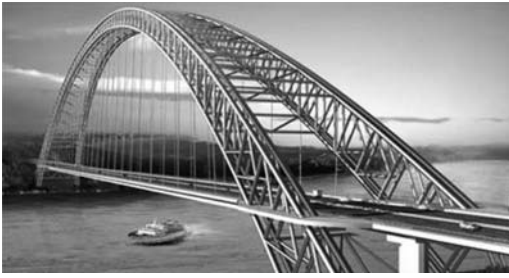
Figure 5. Wu Xia Long River bridge.
