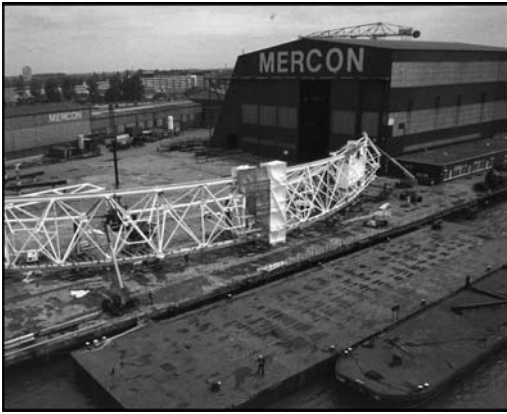
Figure 5. Eye rim segment ready to be loaded onto a barge.
