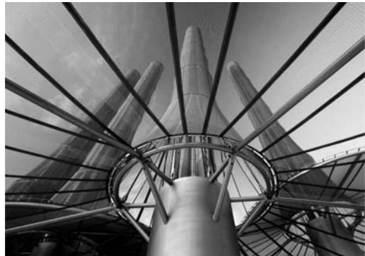
Figure 9. Image of the point where compressions and tensions are transmitted to the lower shaft.
