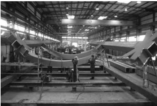
Figure 18. Pre-assembly of diagonals, chords and stars at the workshop.
