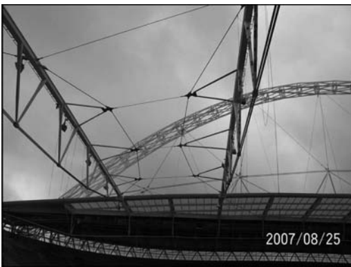
Figure 10. Arch with roof hanging below and over pitch trusses.
