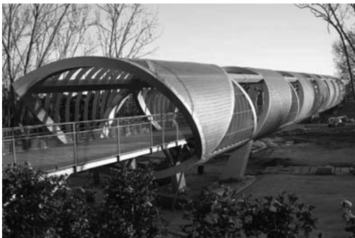
Figure 1. Lateral view of one of the footbridges.
