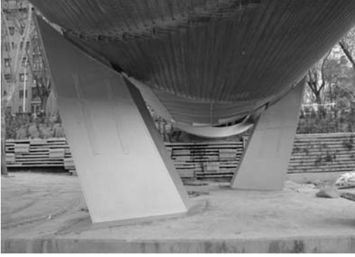
Figure 6. Piers. View from beneath.
