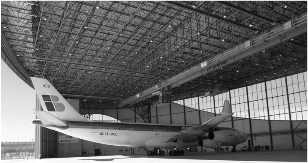
Figure 4. Inside view of the hangar at Barcelona Airport.
