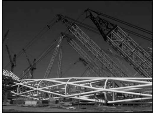
Figure 11. Arch before erection with 5 turning masts in position.
