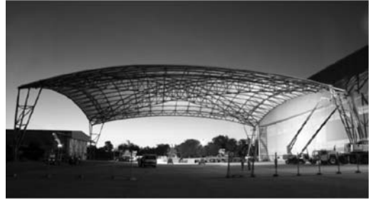
Figure 18. Aircraft hangar with a shell type roofing constructed using intersecting tubular arches.
