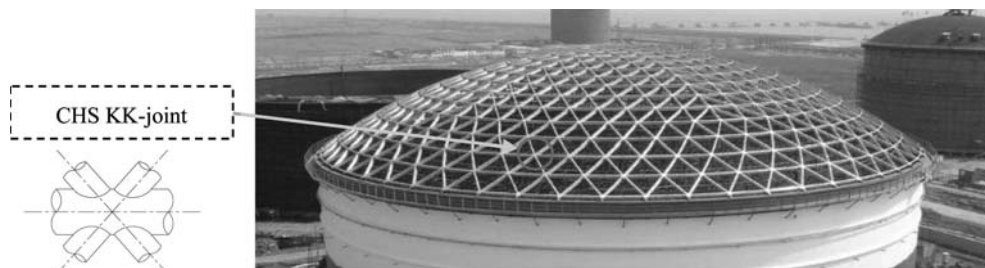
Figure 1. Engineering application of CHS KK-connections.
