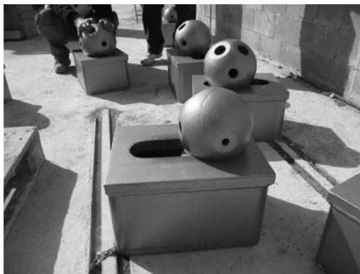
Figure 10. Sliding supports used on the top of the supporting structure.
