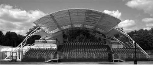
Figure 6. A temporary enclosure with a 25 m clear span.
