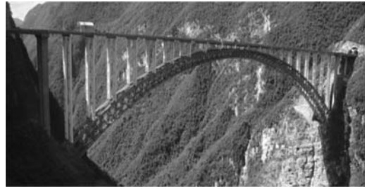
Figure 3. Zhi Jing River bridge.
