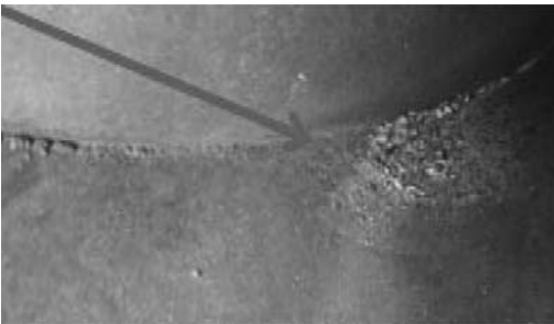
Figure 7b. Undercut and pitting.
