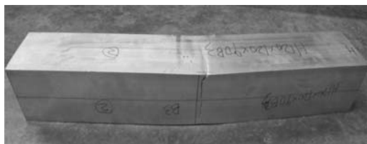
Figure 5. Material splitting on the tensile flange.
