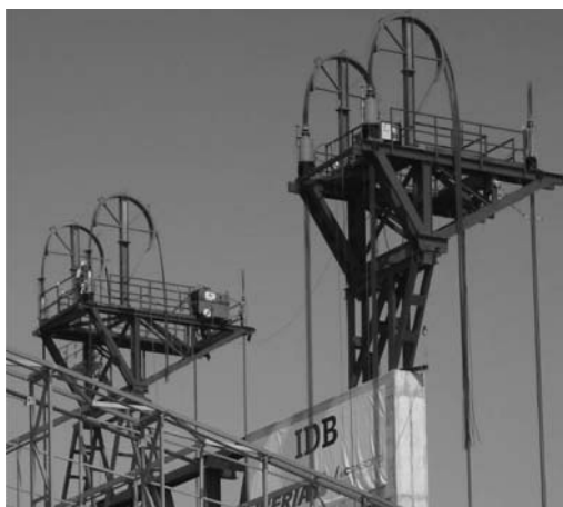
Figure 12. Main hydraulic jacks used for the elevation.
