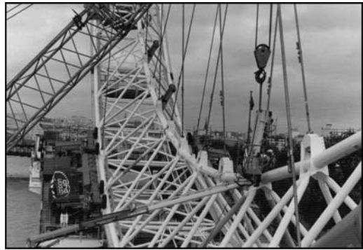
Figure 3. Eye rim interface with drive system.
