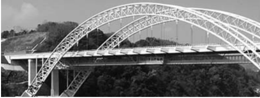
Figure 6. Second Saikai bridge.
