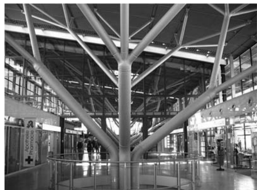
Figure 2. Passengers Terminal, Stuttgart.
