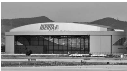
Figure 2. Heavy maintenance hangar in Barcelona Airport.
