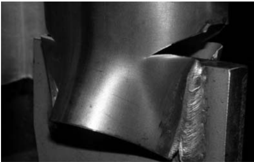
Figure 13. Typical excessive deformation observed at maximum load level.
