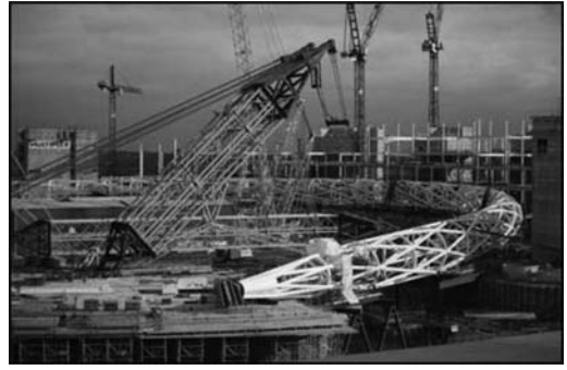
Figure 13. Arch erection with base pinned.
