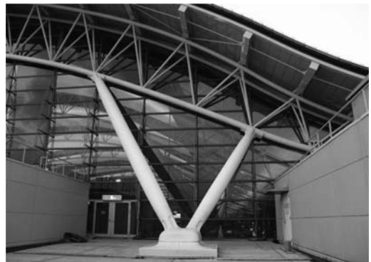
Figure 5. Partial façade Kansai Airport.
