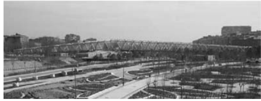
Figure 24. General view of the footbridges and the Arganzuela park.
