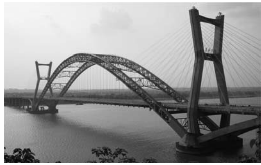
Figure 8. Xiang Jiang Si bridge.
