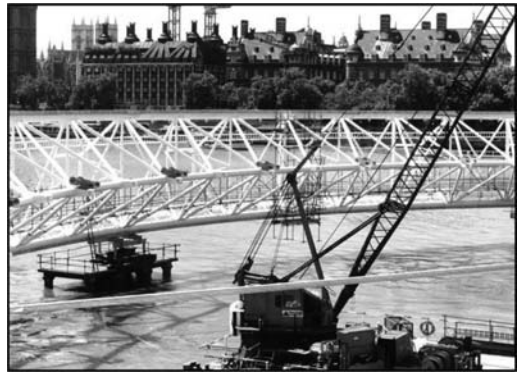
Figure 6. Eye rim temporarily supported above the river.
