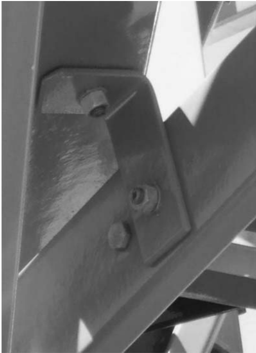
Figure 10. Folded Plate Connection (note head of bolt for connection on far side).
