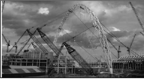
Figure 16. Arch going ‘over the top’.
