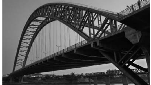
Figure 4. Yong River bridge.
