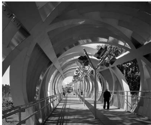
Figure 2. Inside view: Pedestrian and cyclist lanes.
