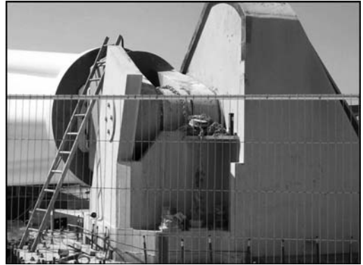
Figure 14. Erection pin at arch base.
