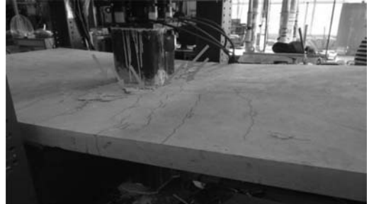
Figure 10. Fine cracks near the column.
