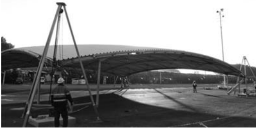
Figure 20. Erecting a shell structure made using post-tensioned LSB members without cranes.
