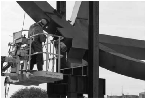
Figure 22. Welding of a diagonal to a star.
