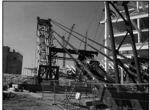
Figure 15. Strand jacks for pulling up turning masts.
