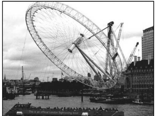
Figure 7. Eye erection.
