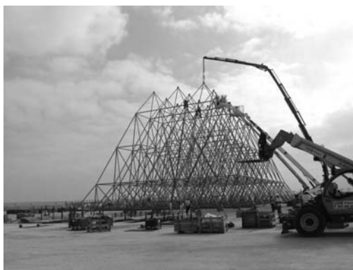
Figure 11. Central part of the arch assembled on ground.
