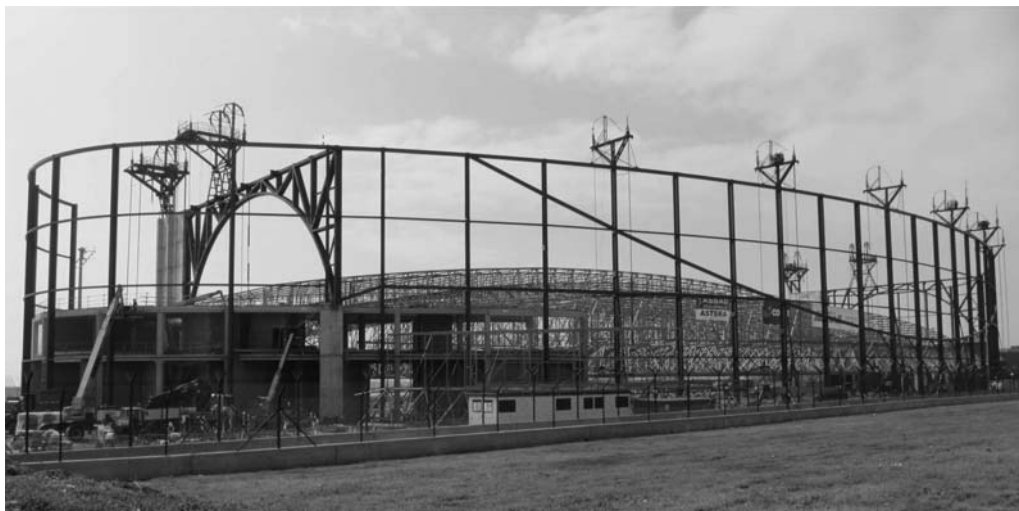
Figure 13. General view of the structure during lifting.
