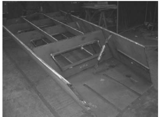
Figure 19. Pier under construction at workshop.
