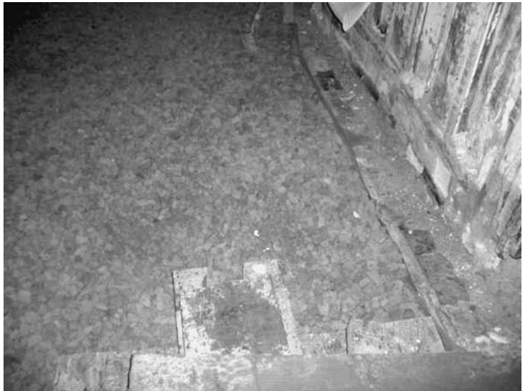
Photo 7.32b Limecrete floor technology – a newly laid foamed glass sub-base
