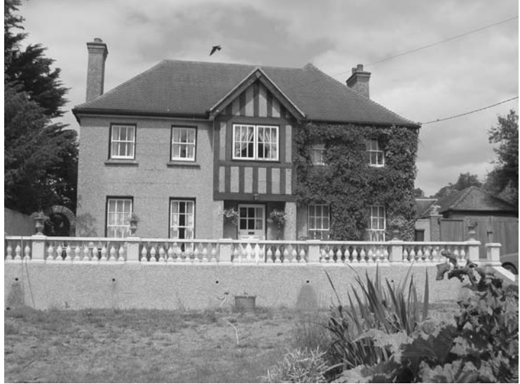
Photo 5.1 Mock timber framing facing into the elements was always going to be problematic
