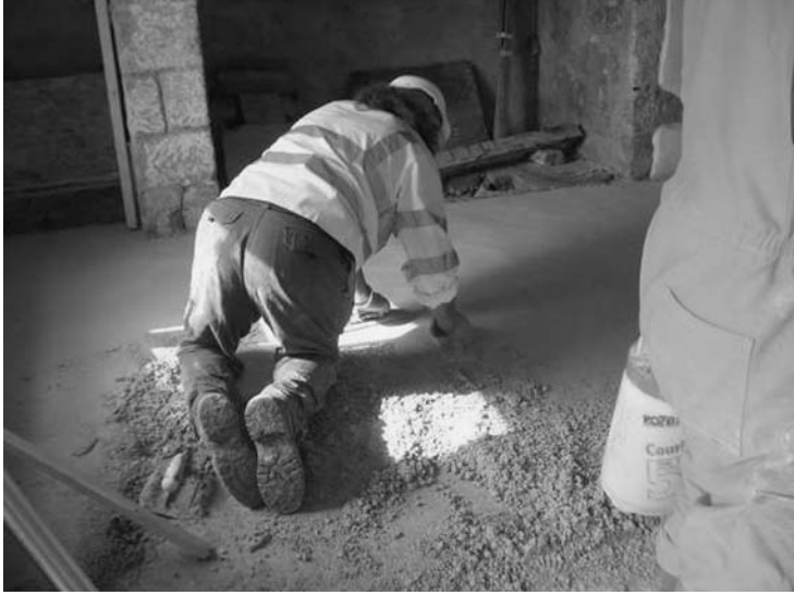
Photo 4.2 A limecrete floor being laid
