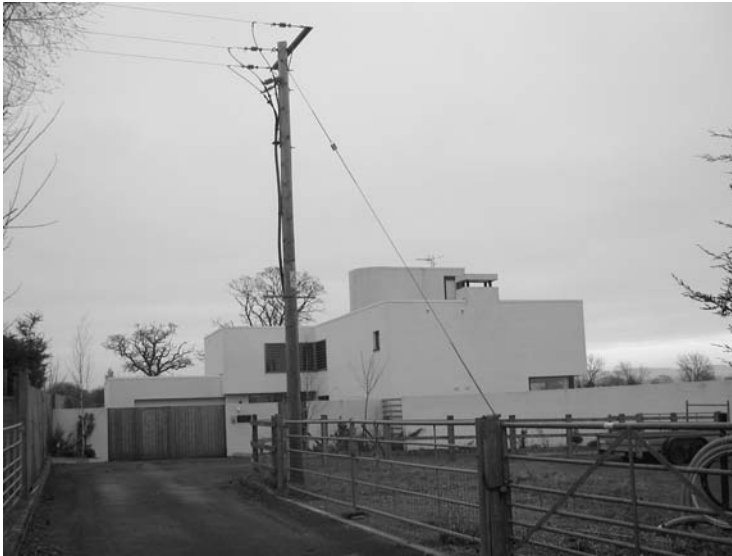
Photo 1.32 A brand new Modern movement inspired sustainable house
