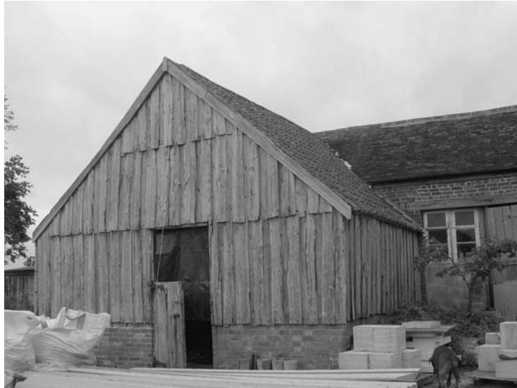
Photo 3.24 A Dorset farm building with vertical boarding with cover strips
