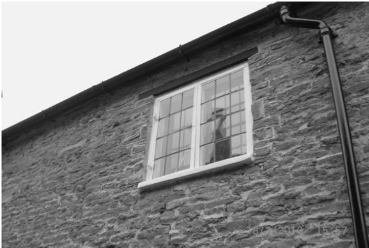
Photo 3.7 Random uncoursed stonework
