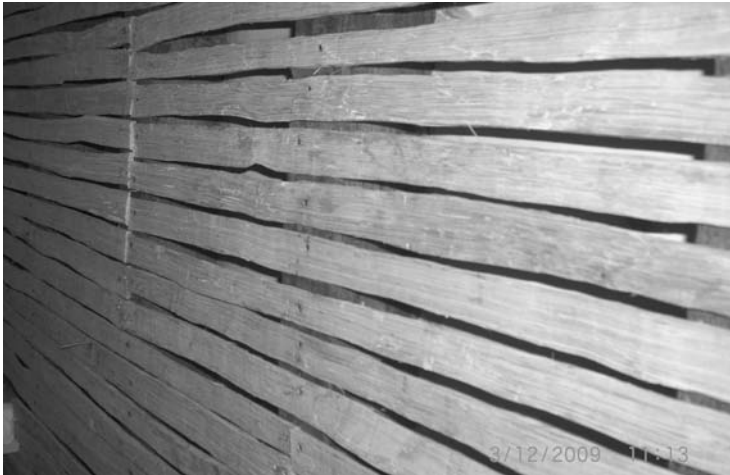
Photo 7.15 Battens for internal lime plaster on ceilings
