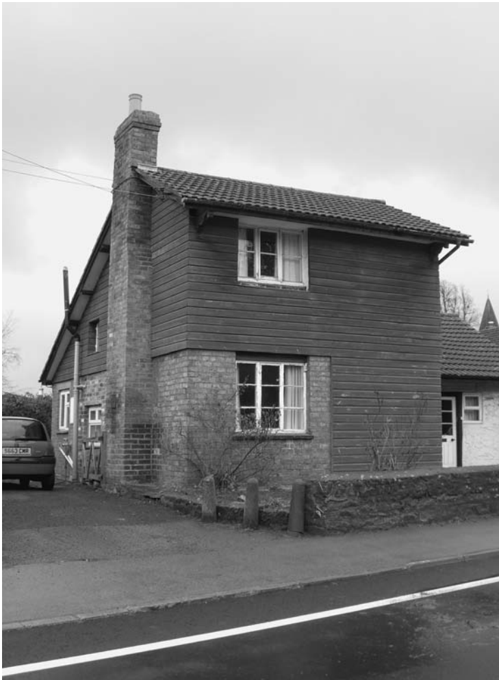
Photo 4.4 External boarding and insulation may not be out of place on a simple brick cottage
