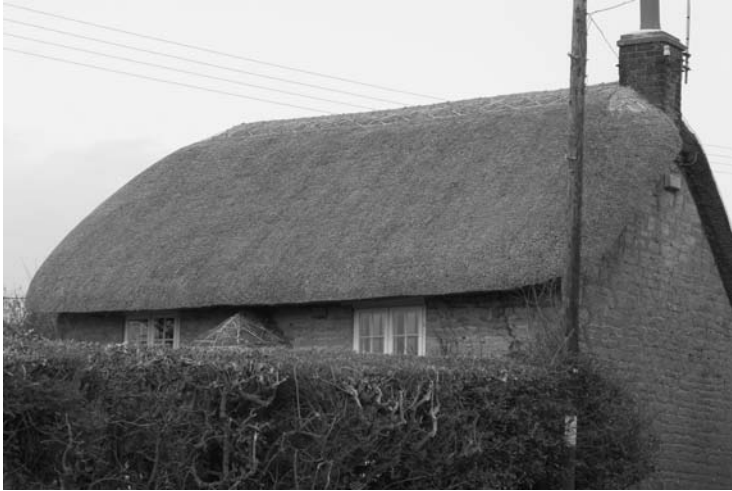
Photo 3.27 A recently repaired traditional combed wheat thatch with liggers
