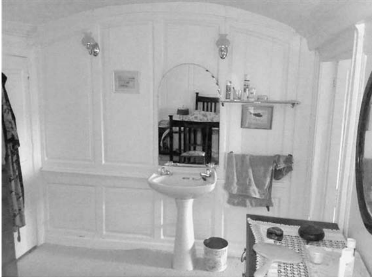
Photo 6.16 A former 18th-century panelled bedroom in use as a bathroom with all the attendant problems that will be caused to the fabric by condensation
