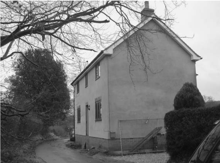
Photo 2.10 Blockwork replacement building for the rejected cob house
