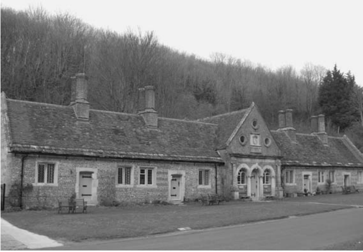
Photo 5.21 Almshouses in Milton Abbas, Dorset, now have a heat ventilation recovery system to remove condensation and improve air quality
