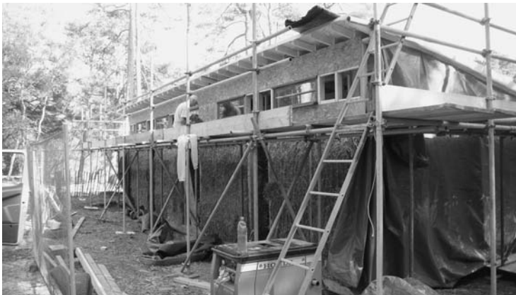
Photo 6.9 Straw bale construction nearing completion (photo © Rob Buckley)
