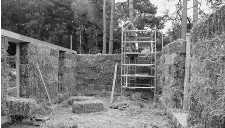
Photo 6.8 Straw bale in construction (photo © Rob Buckley)
