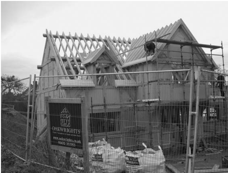
Photo 3.17 Traditional post-and-truss framing employed in new build
