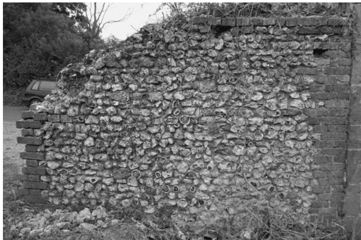
Photo 3.12 A rare survival of untouched flint walling
