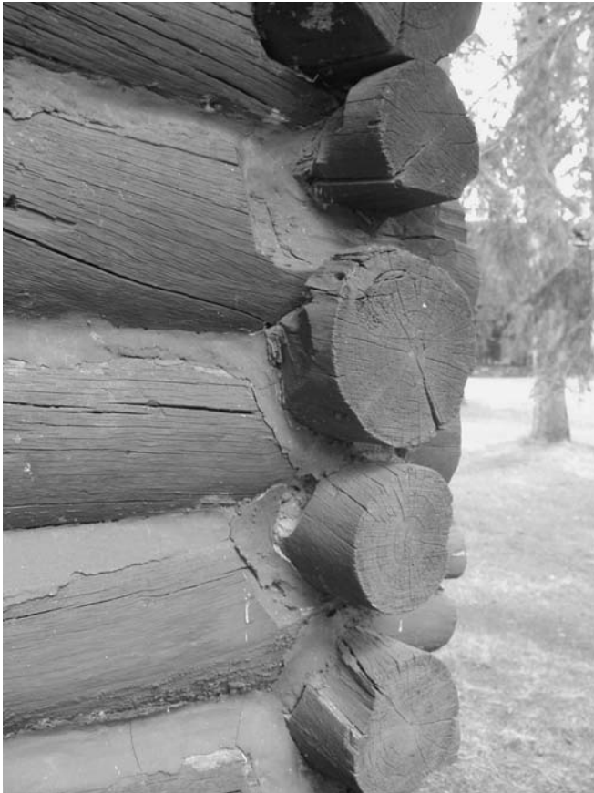
Photo 2.41 Interlocking half lap joint on the corner of a log cabin reconstruction at Banff, Canadian Rockies
