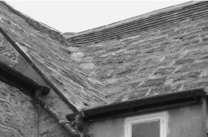
Photo 3.32 A swept valley in stone tiles
