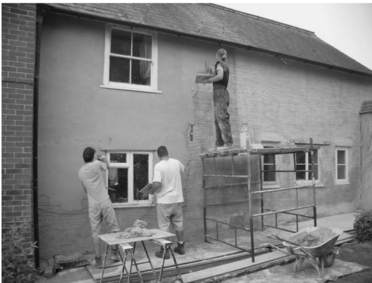
Photo 4.26 Lime rendering being applied (photo © Rob Buckley)
