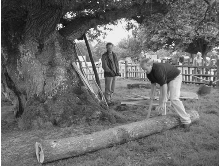
Photo 2.33 Processing a beam – side axing commences to remove the sapwood
