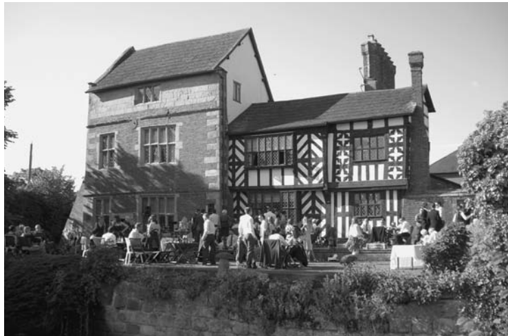
Photo 2.39 Quatrefoil and diagonal bracing showing use of smaller pieces of timber by about 1600
