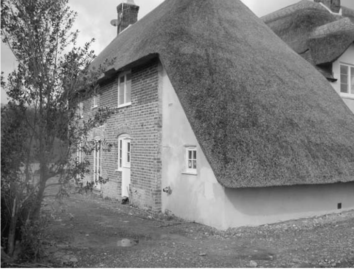
Photo 1.4 Long, low, sloping thatched roof deliberately contrived to protect the rest of the building from adverse weather conditions.
