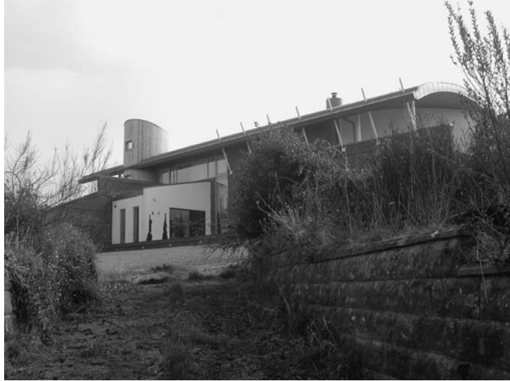
Photo 6.25 Purpose-built passive stack ventilation on a sustainable construction
