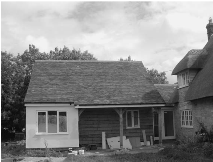
Photo 5.12 A link detached extension is often the only means of obtaining the live-in kitchen currently so desirable
