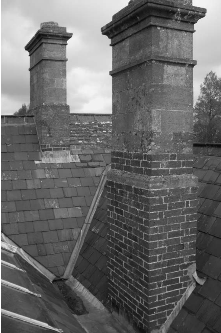
Photo 3.5 Fine ashlar work used on the chimney of a country house
