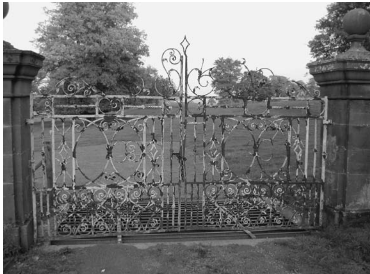
Photo 2.50 A wrought iron gate c.1820 in urgent need of repainting and repair
