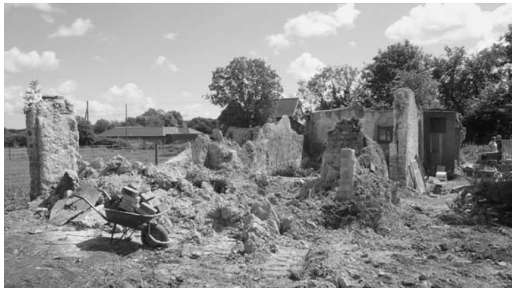
Photo 2.5 Cob building returning to earth (photo © Rob Buckley of DCRS)
