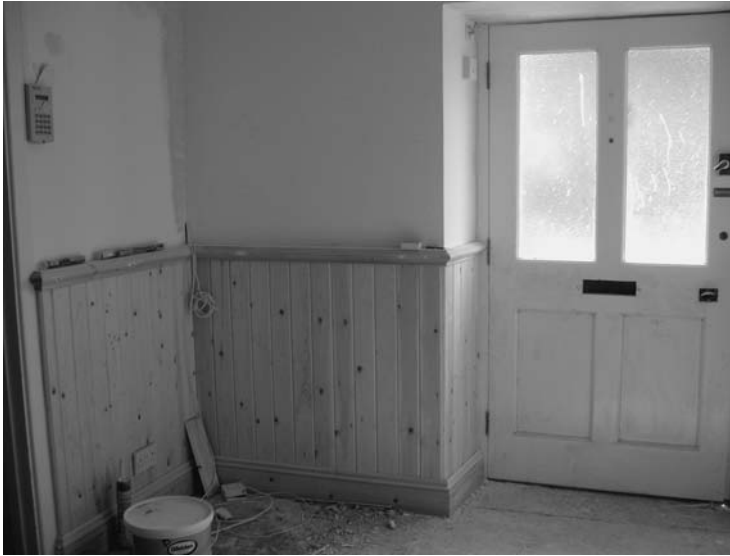
Photo 4.27 New matchboarding being re-applied to a traditional stone building
