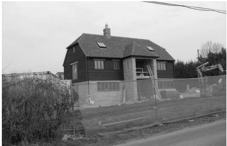
Photo 2.26 The replacement, doubtless sustainable but then so was the original
