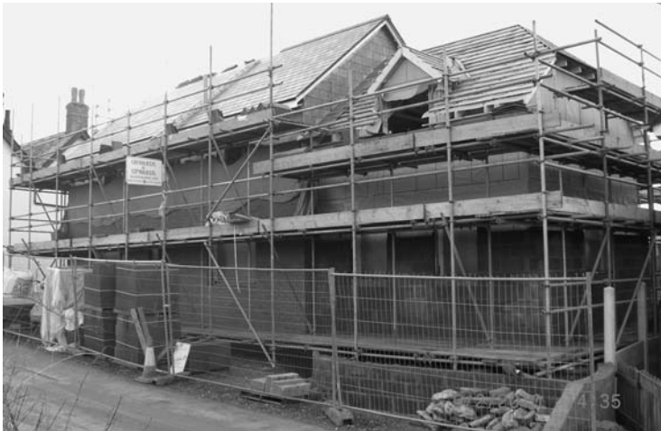
Photo 3.18 A modern timber frame under construction
