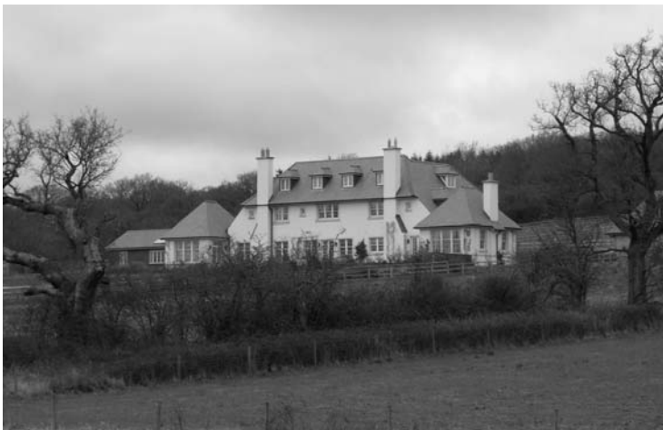
Photo 5.13 A large-volume new build in open countryside has a higher ventilation heat loss rate
