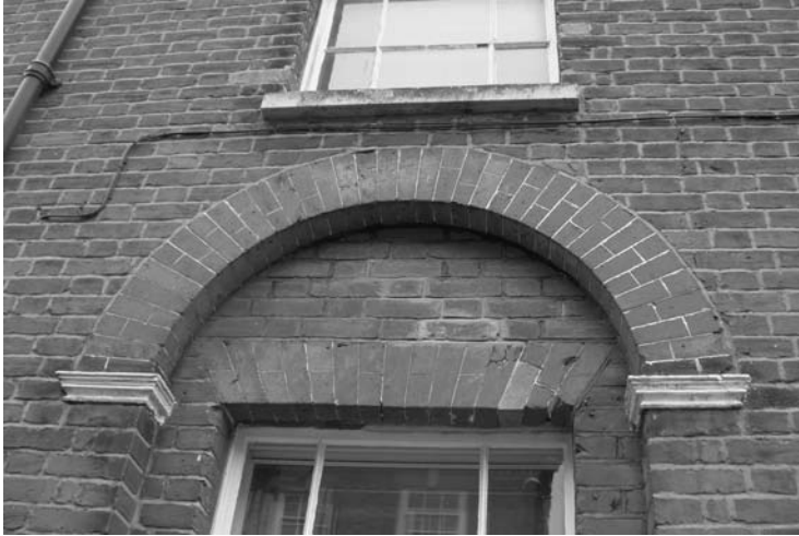
Photo 2.17 A traditional rubbed brick arch
