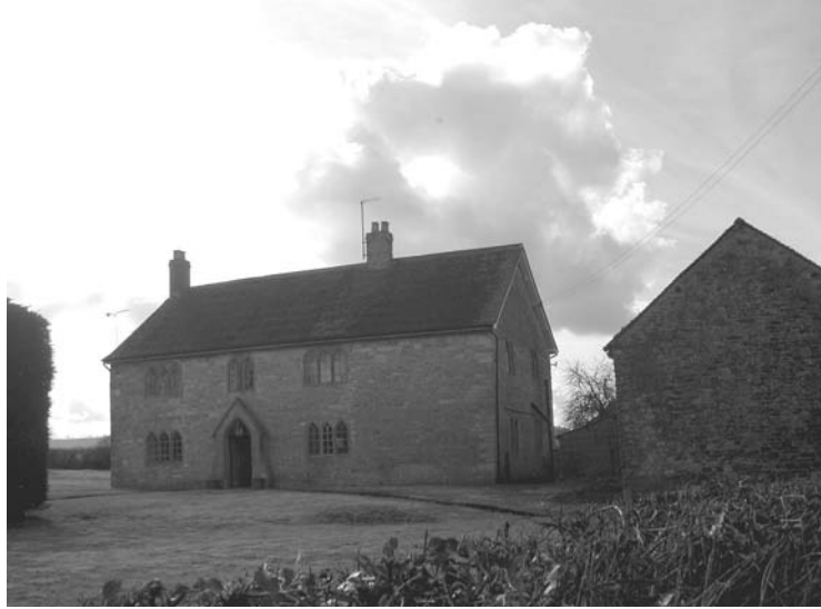
Photo 6.15 A Dorset house and barn about to be joined together to form a major complex, an exercise which will require stringent satisfaction of the Building Regulations
