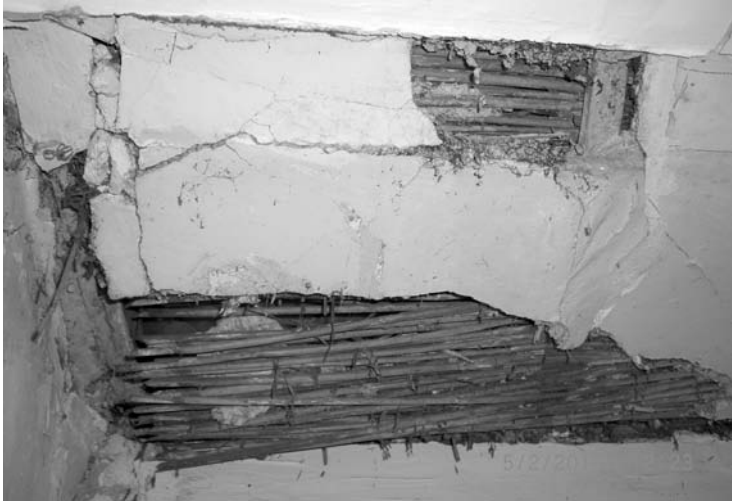
Photo 2.46 Plaster on reed
