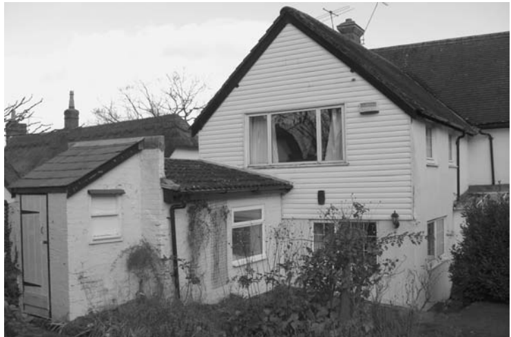
Photo 2.55 Unfortunate plastic cladding and UPVC windows in a traditional building are not sustainable
