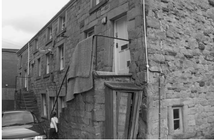
Photo 1.23 Workers' housing in Buxton, Derbyshire
