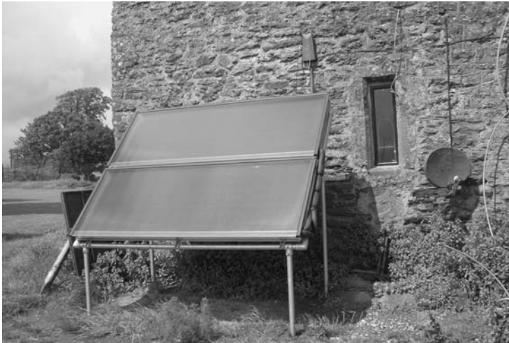
Photo 3.38 A discrete location for solar panels on a medieval building
