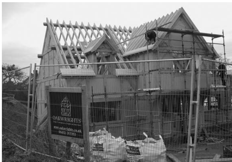
Photo 6.13 New timber framed building in Herefordshire during construction
