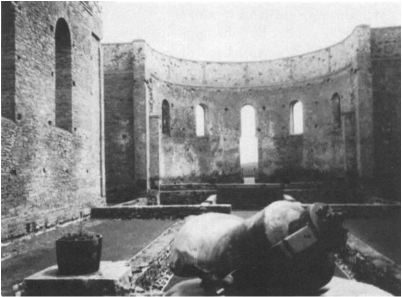
The Ruins of St. Raphael are all that is left of a once grand old church. The walls still stand just as the faith of our forefathers has stood down through the years.
