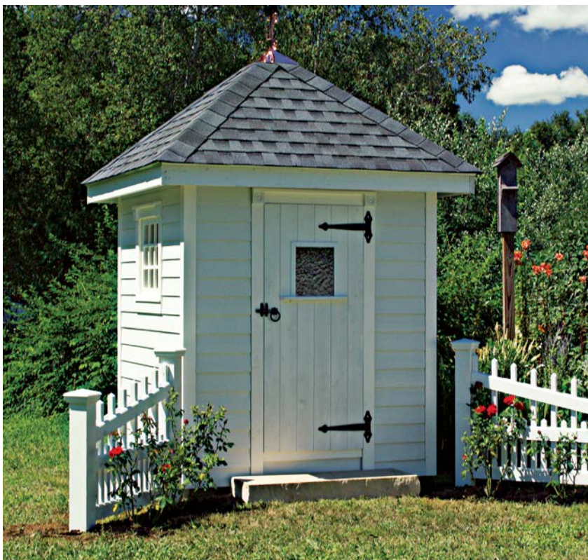
This diminutive garden shed features a distinctive hip roof, which is easily recognized by its four sloping roof planes.
