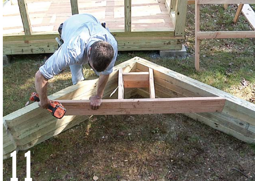
Frame each gable-end truss for a vent. Nail the header between the vertical nailers and attach the sill. Then nail the assembled frame to the rafters.
