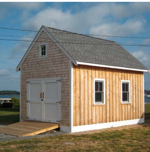
This spacious seaside shed features two types of siding: white cedar shingles on the gable-end walls and board-and-batten siding on the sidewalls.
