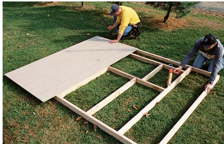
Textured plywood siding comes in large sheets for quick, easy installation. And it can be nailed directly to the wall framing; no sheathing needed.
