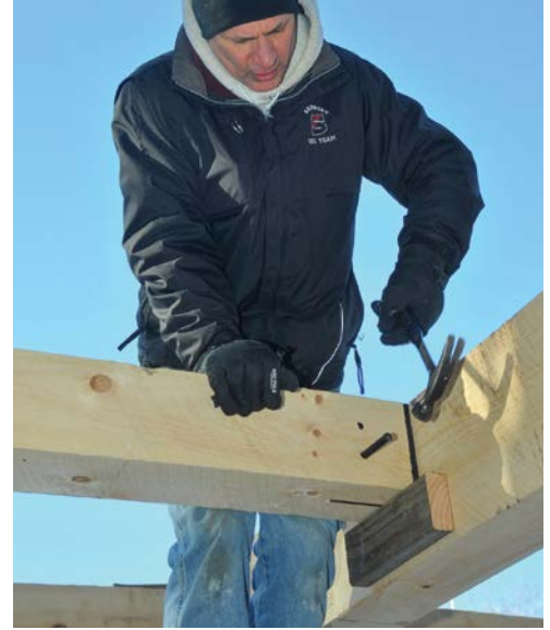
The beam is securely locked in place with two 1/2-in.-dia. metal pins, which are driven into holes bored through the beam and connector.
