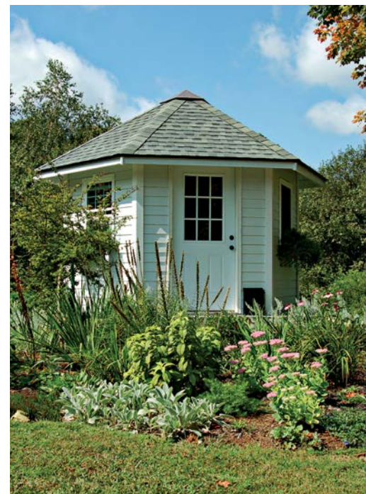
This hexagonal outbuilding is topped with a hip roof that extends past each of the shed's six walls, creating an overhanging eave.
