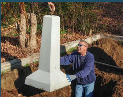
A. Ready-to-install precast-concrete piers consist of an extra-wide base (footing) and tapered column. Lower the piers into the holes with a backhoe.
