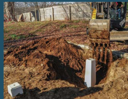
C. Backfill around each precast pier with soil. The piers should protrude above grade by at least 4 in. to allow air to flow beneath the shed.
