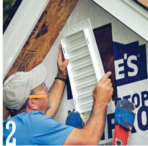
2 Place the mounting base of the louvered vent into the hole at the top of the gable-end wall. Fasten the PVC base with roofing nails.
