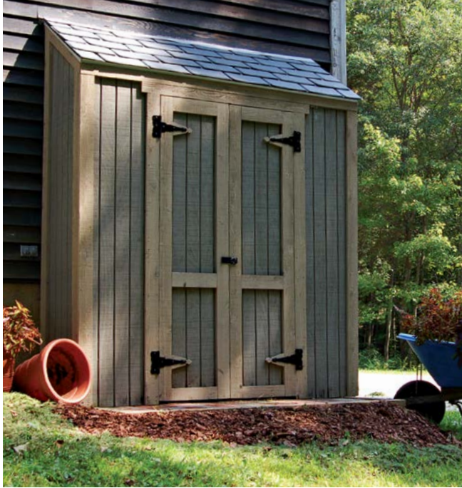
A shed roof has a single sloping roof plane, which makes it ideal for lean-to sheds that are built up against another structure.
