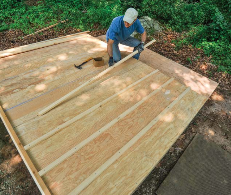
A quicker way to create board-and-batten siding is to sheathe the walls with rough-sawn plywood and then nail on equally spaced wood battens.
