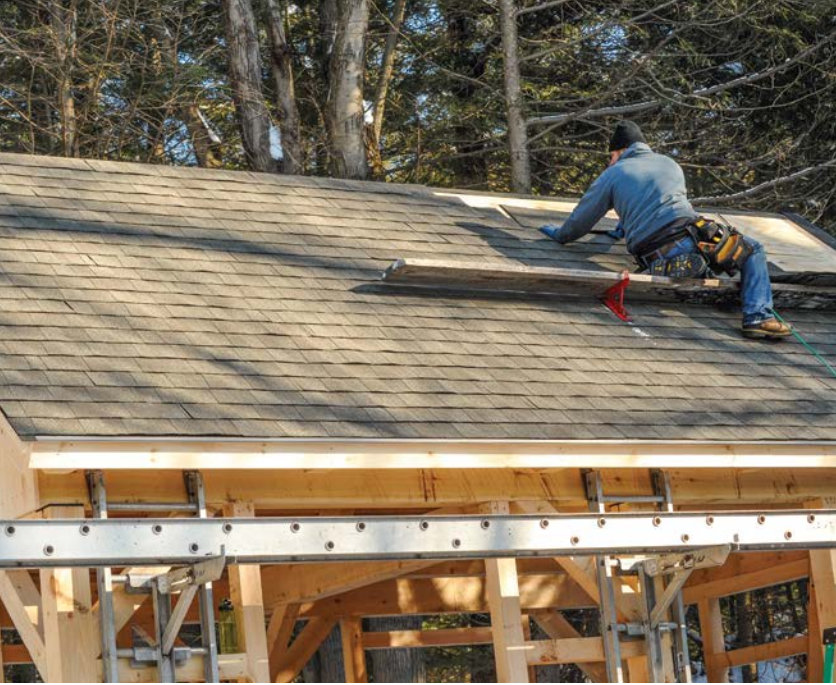
Architectural-style roof shingles are thick and heavily textured. The roof shown here is designed to look somewhat like weathered wood.
