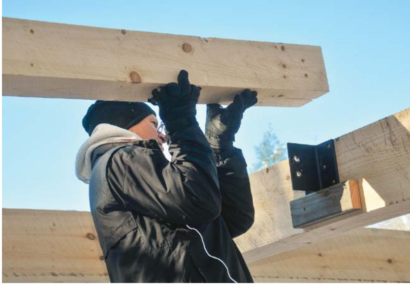
Metal T-Rex™ connectors greatly simplify post-and-beam construction. The protruding flange fits into a slot cut in the end of the beam.
