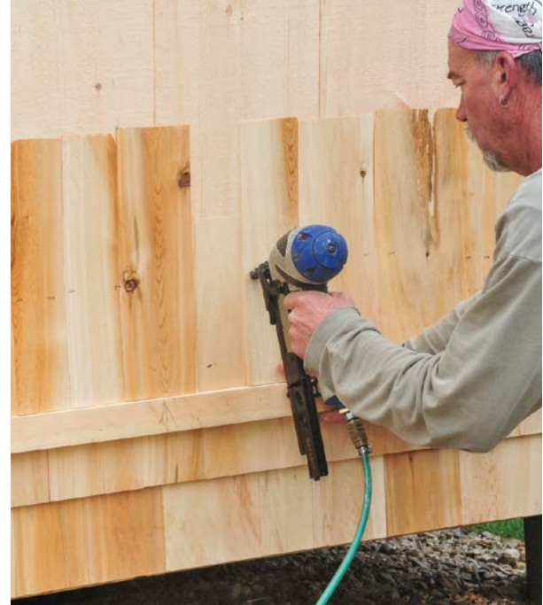
Shingles are fastened to the walls in overlapping courses. To ensure a weatherproof surface, all vertical seams must overlap by at least 1 1/2 in.
