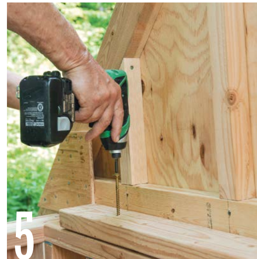
Secure the truss to the top of the gable-end wall by driving 3-in. screws down into the top wall plate; space the screws 12 in. apart.
