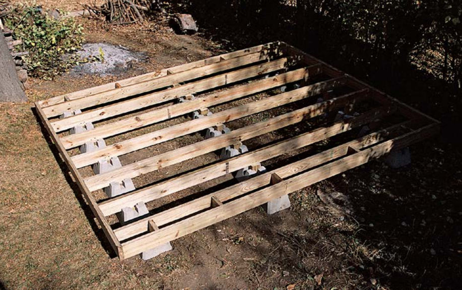
Precast-concrete pier blocks , laid out in parallel rows, provide a quick and easy way to support the shed's pressure-treated floor frame.
