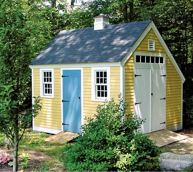
A saltbox roof adds a bit of Colonial charm to this 12-ft. by 14-ft. storage shed. The rear roof plane is slightly longer than the front roof plane.
