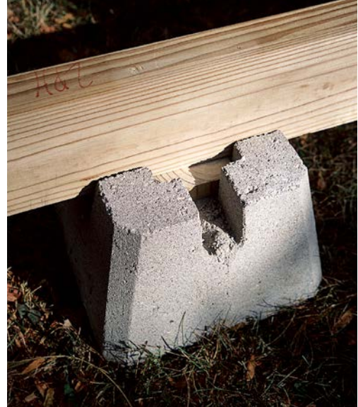
Each pyramid-shaped concrete pier block has slots molded into its top surface, which are sized to accept a 2× floor joist.
