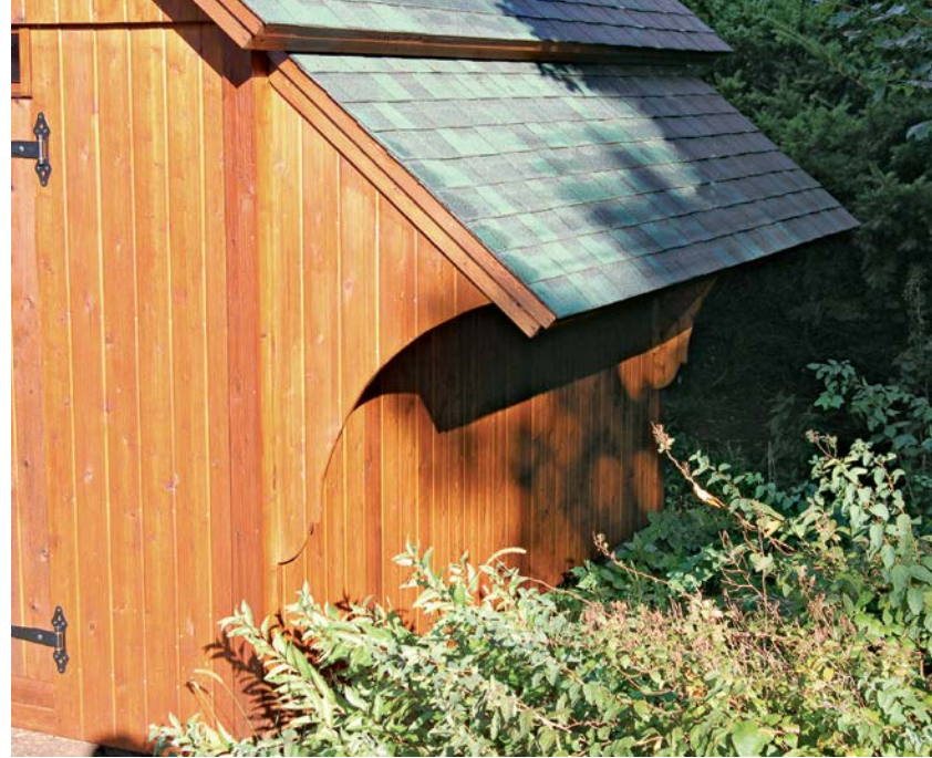
This cleverly designed saltbox shed has a rear wall that's recessed 2 ft. beneath the roof overhang to create a readily accessible storage nook.
