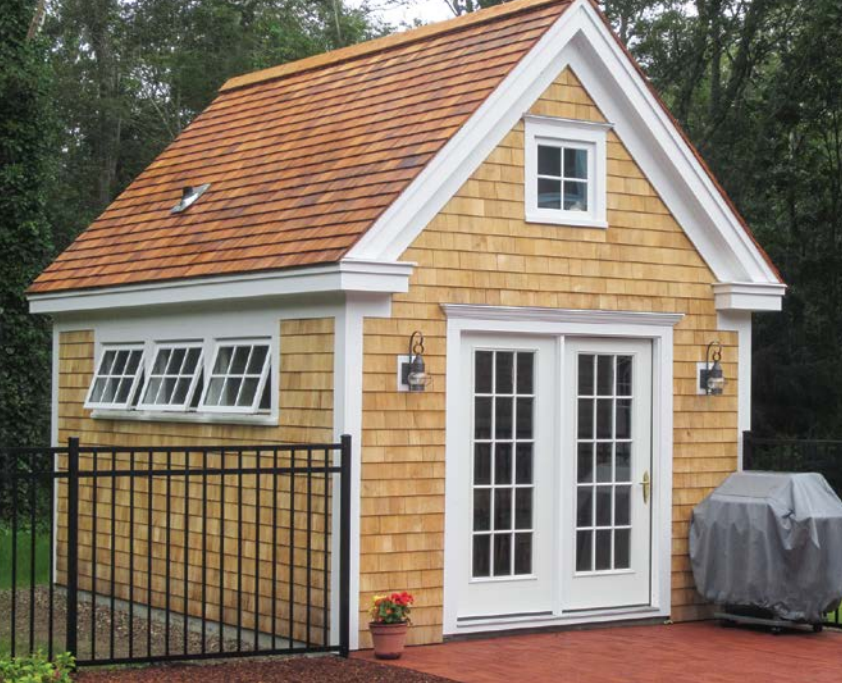
This beautiful pool cabana is festooned completely in wood shingles: red-cedar shingles on the roof and white-cedar shingles on the walls.
