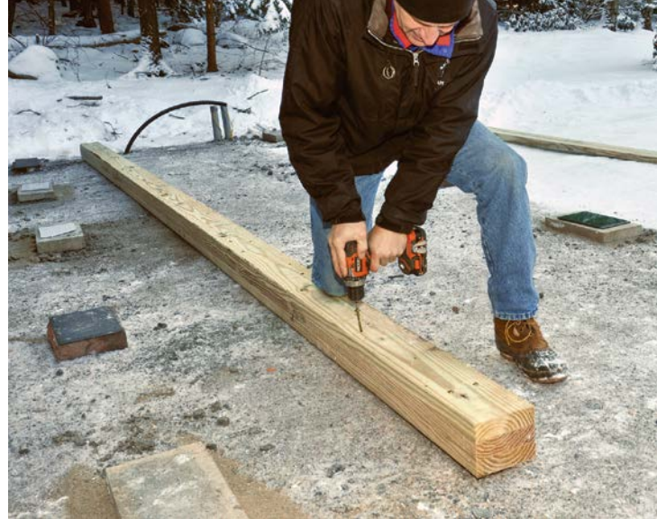
Skids can be cut from solid timbers , such as 6×6s or 8×8s, or you can make them by fastening together three long 2×6s or 2×8s.
