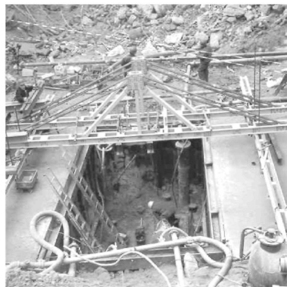
Figure 15 Testing set up for the wooden pile loading test
