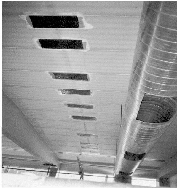
Figure 8 Reinforcement of drilling holes
