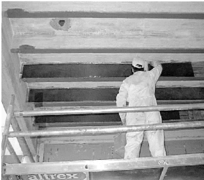
Figure 3 Application of the CFRP sheets
