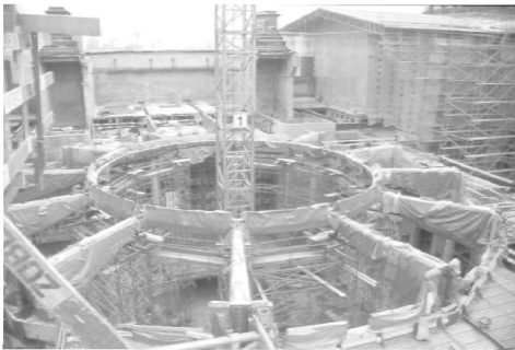
Figure 16 Erection of assembly room ceiling
