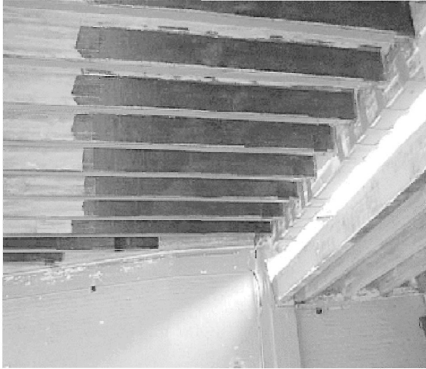
Figure 4 Hybrid strengthening of ribbed floor slab
