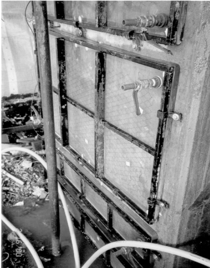
Figure 2 Cassette shutters which contain titanium mesh anode and electrolyte
