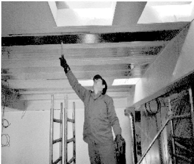
Figure 7 Impregnation of CFRP-sheets
