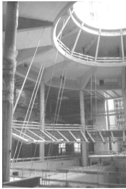
Figure 17 Ceiling of assembly room from inside during construction:
