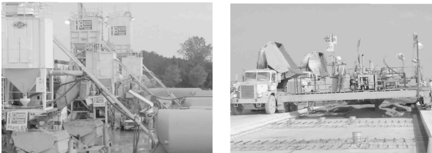
Figure 5 Batching and Placement of Concrete
