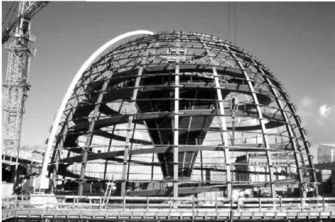
Figure 18 Dome during erection
