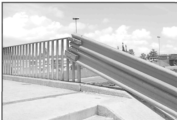
Figure 1 Guardrails used to repair balustrades of Bridge B488 over the N3
