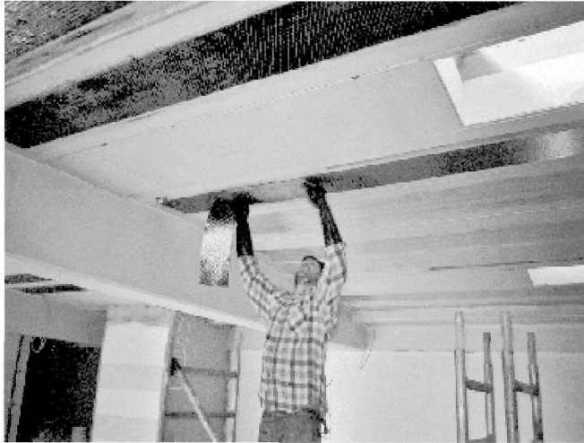
Figure 6 Application of CFRP-sheets
