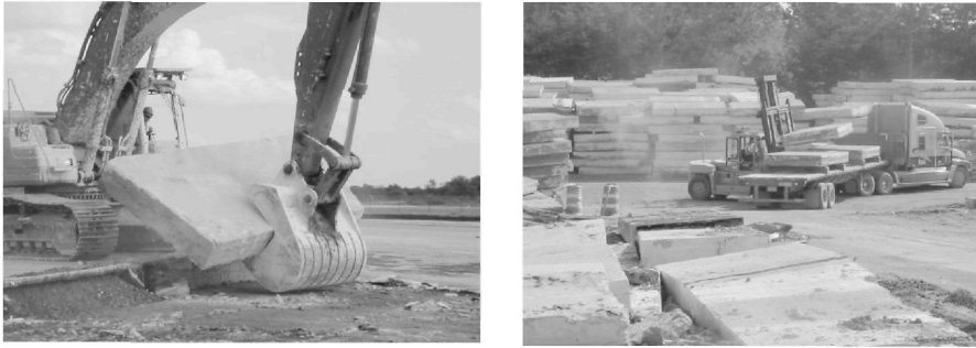
Figure 4 Removal of Existing Pavements
