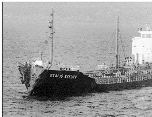
Figure 1 Overall view of vessel with damaged bow
